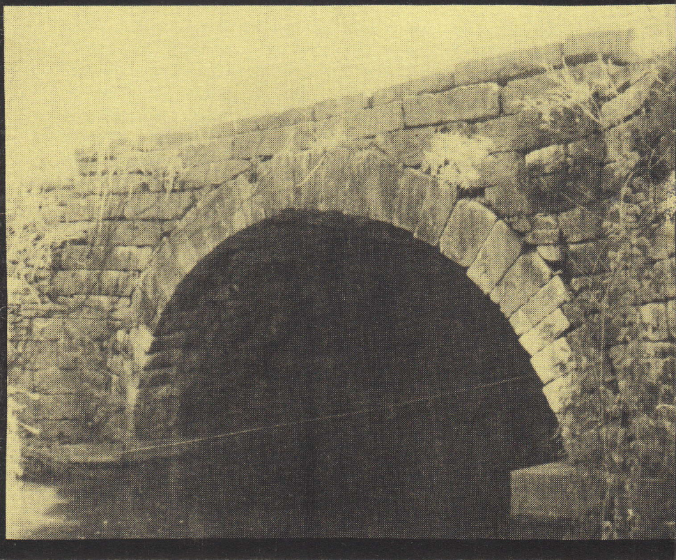
Culvert No.100 over Burnett's Creek
