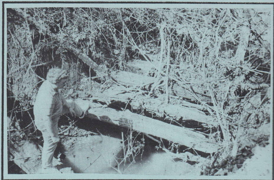
Stan Schmitt doing field research on the Cross-Cut Canal. Lock# 50, timber crib, similar to Lock# 43 in this issue. Shown are the remains of the 36' foundation timbers. (a la Gronauer Lock).
