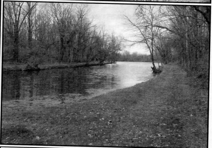
Center: Composite Lock 50 with cut stone entrance and rubble stone chamber that once was lined with wood. Bottom: A dam was built across the Hagerstown Extension to create Scout Lake pictured here.
