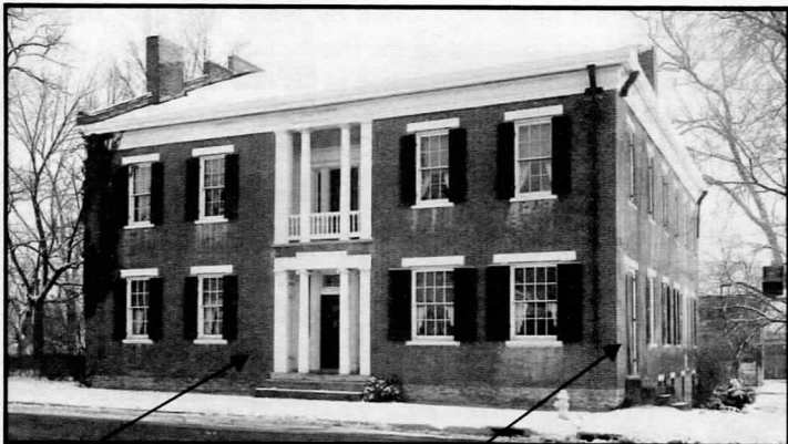
Home on east side. Business Entrance on west side near river. The Conklin-Montgomery House in Cambridge City, Indiana
