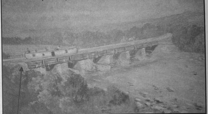
Photos of aqueduct painting and 5th street abutment - Bob Schmidt
