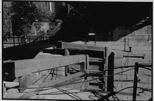
New lock gates Photo by Bob Schmidt June 2014
