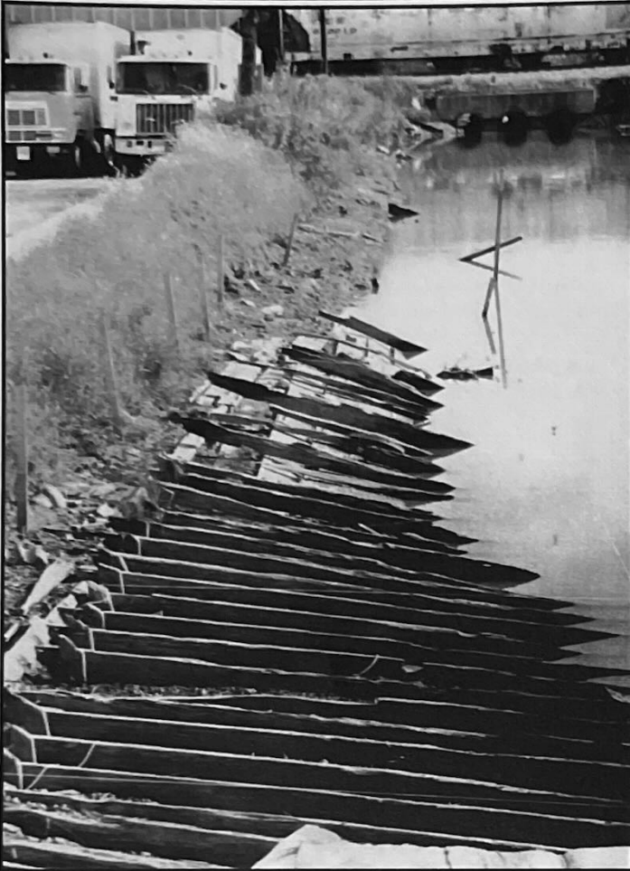
The bottom planks of the Marguerite I are seen above in the Miami & Erie Canal in Delphos, Ohio.
