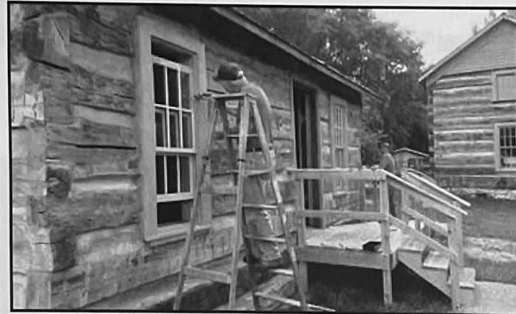
Tom Peters trimmed the recently installed windows.
