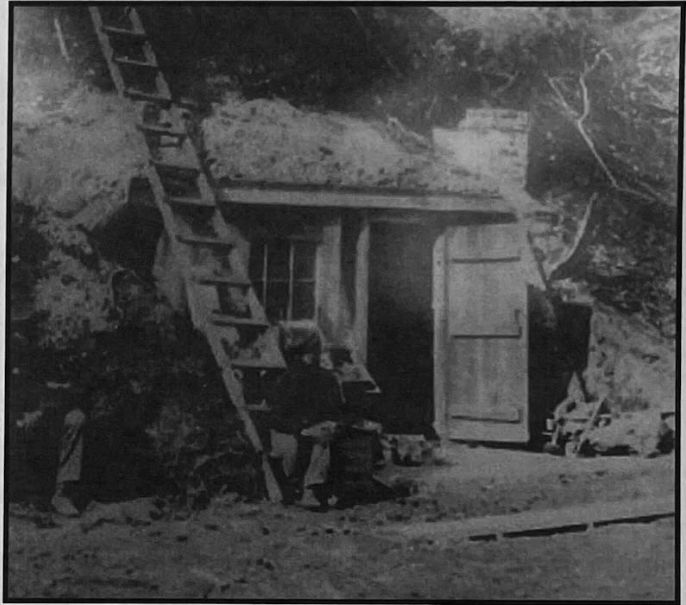
Above: 1864 photo of USCT picket post at the Dutch Gap Canal on National Park signage from Library of Congress.
