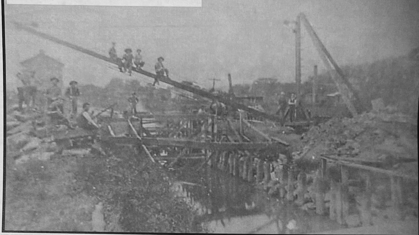
Building the Ohio & Erie Canal in the area of Clinton, Ohio
