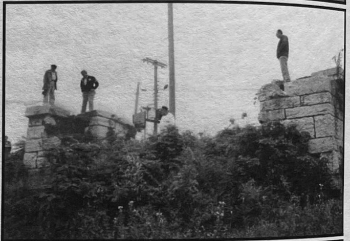
Top: Aqueduct No. 5 is shown in a painting by Wils Berry in the Cass County Historical Museum. Photos by Bob Schmidt Bottom: On a tour CSI members stand on the south abutments of Aqueduct No. 5. The trough went between these structures.
