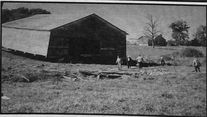
1. Crossing farm fields with the warehouse 2. Crossing a highway 3. Moving electrical lines 4. Bridge built over ditch by Norman Skinner Photos by Norman Skinner
