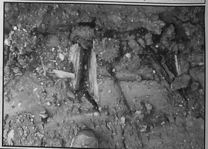
Timbers under Lock One South—photo by Preston Bartlett
