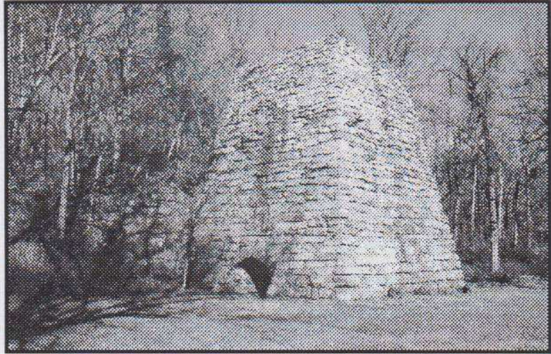
Illinois Iron Furnace has been reconstructed as a memorial. Photo by Bob Schmidt
