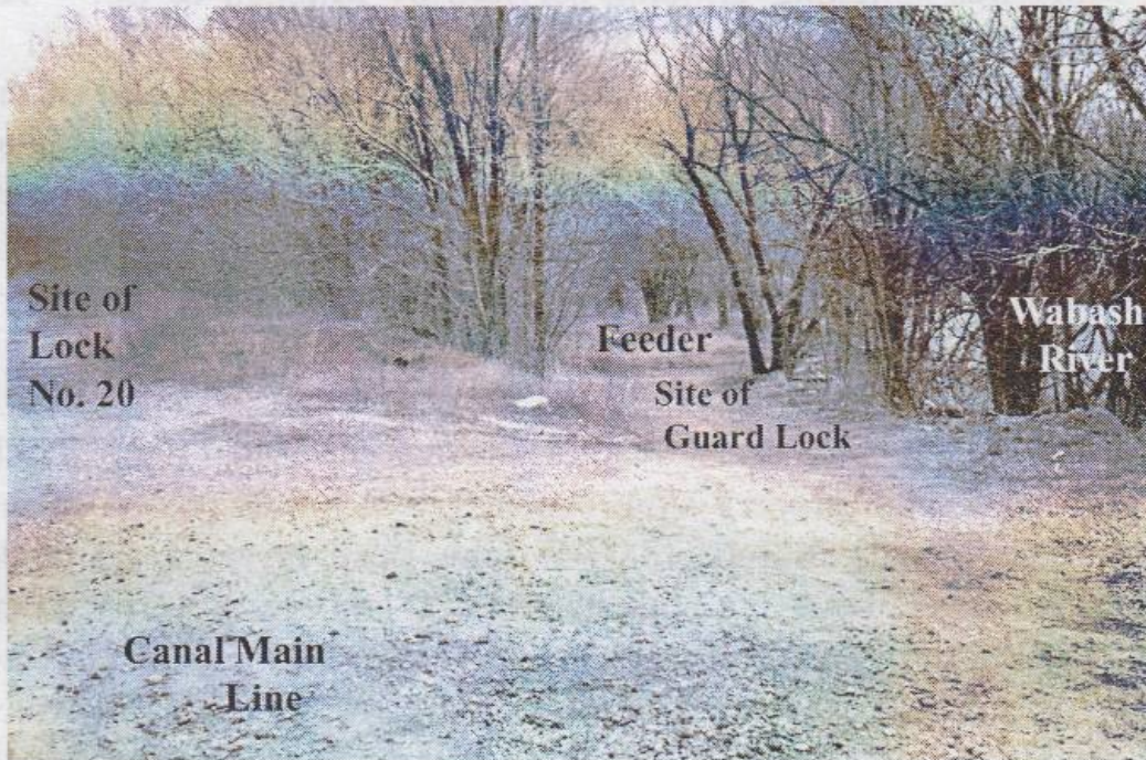
Present location where Wabash River Dam No. 3 once replenished canal water from the river through a feeder channel, which joined the main line at a guard lock below Lock No. 20. Photo in author's collection.
