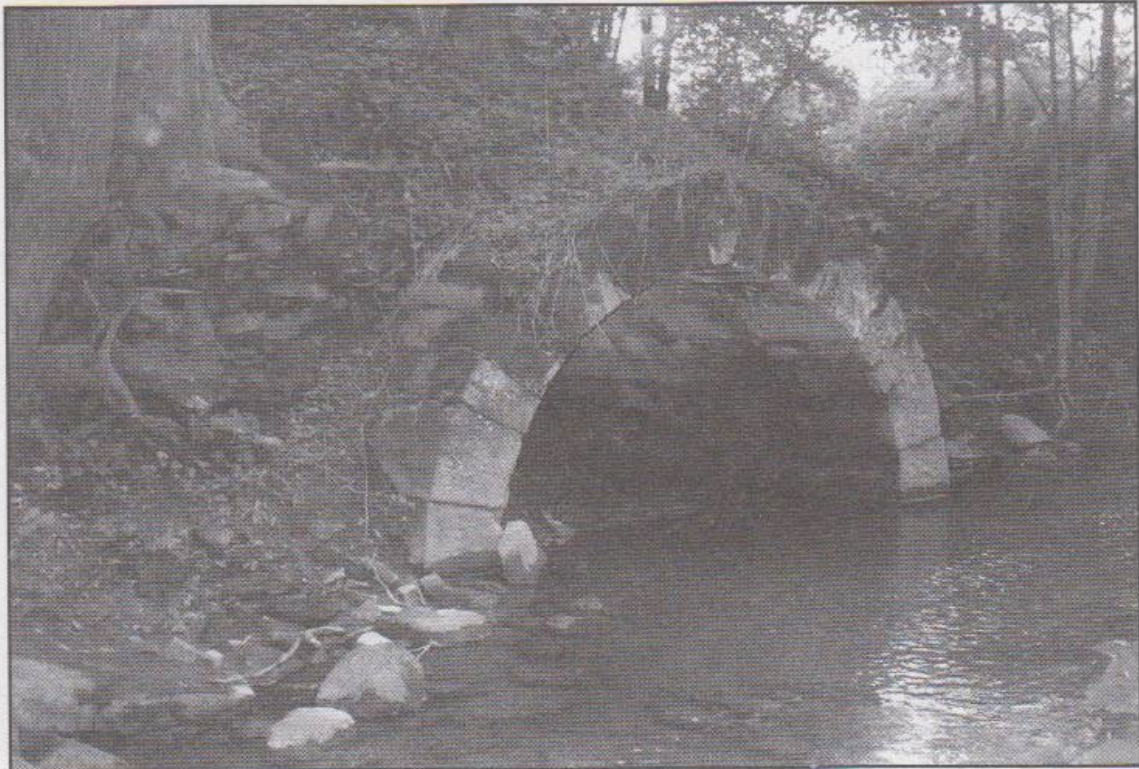
Cottonwood Creek stone arch designated Culvert No. 88 was made of stone from the Georgetown Quarry.
