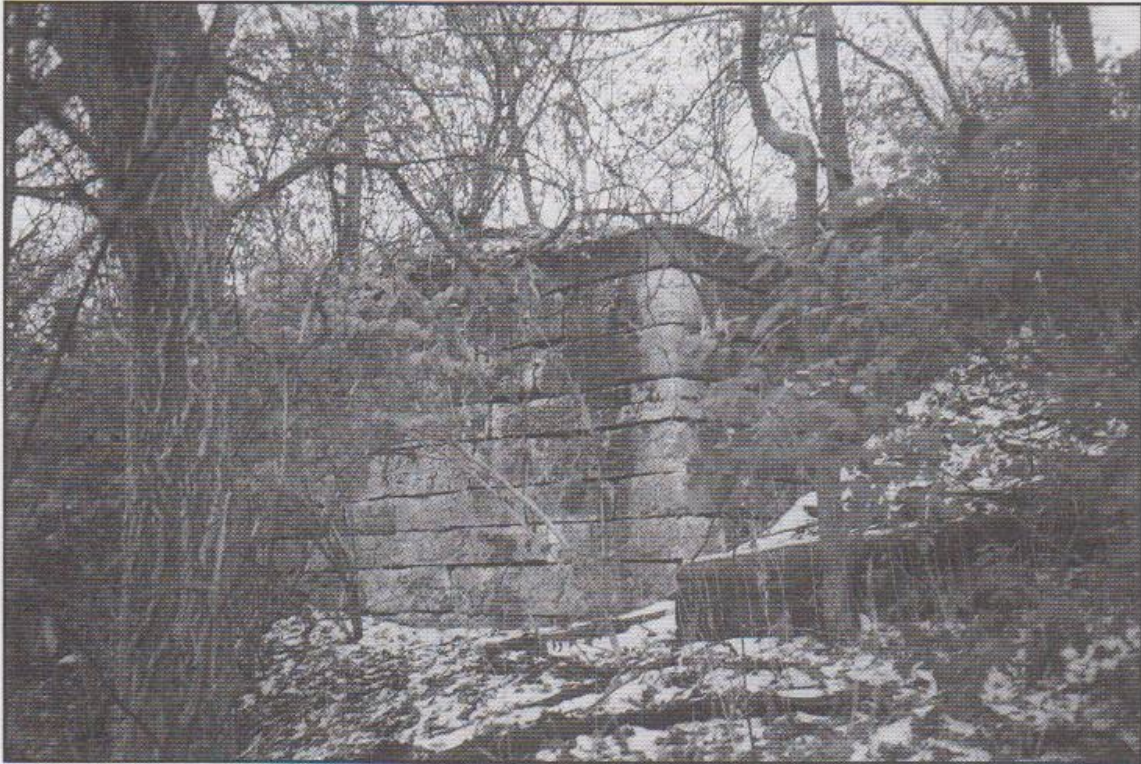
Wildcat Creek Dam south abutment stands today among large cottonwoods and wild underbrush.
