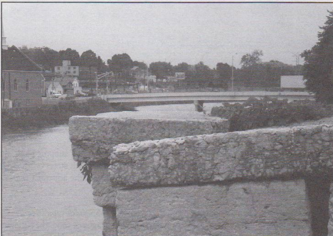
Aqueduct stone abutments on the south bank of the Eel River.
