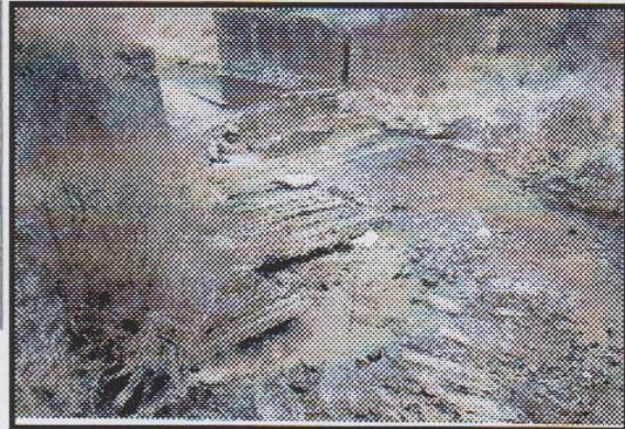
The cut stone remains of the Aboite Creek abutments are seen on the left and top center of this photo with the timber remains and some stone from the piers in the creek. Photo by Bob Schmidt 1997
