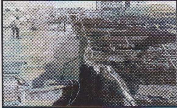
Above: The North American trailer served as storage for equipment and a sprinkling system kept the lock wet. Below: The huge timbers within the cribs still had bark on them. Photos by Patricia Derrow
