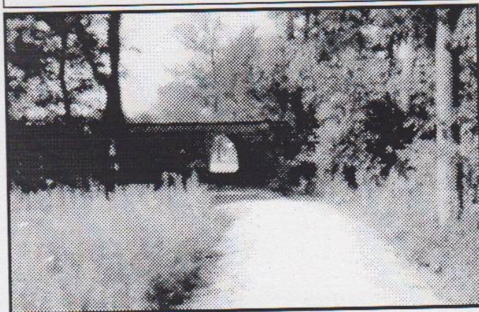
A tunnel was built under the railroad track. Photo by Bob Schmidt
