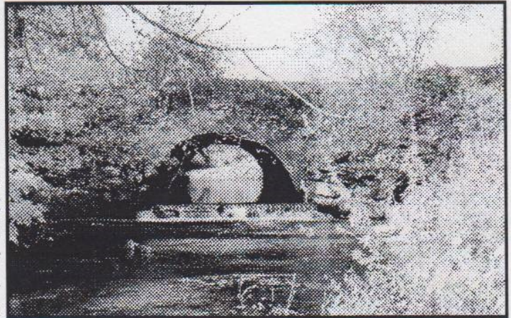
Burnett's Creek Culvert #100 Photos by Bob Schmidt
