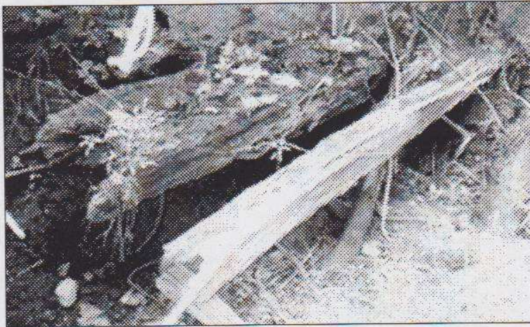
Culvert No. 52- Notebook III , p. 18
