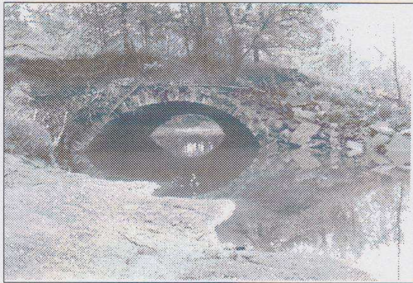
Stone Arch Culvert No. 45 over Silver Creek Notebook I p. 89
