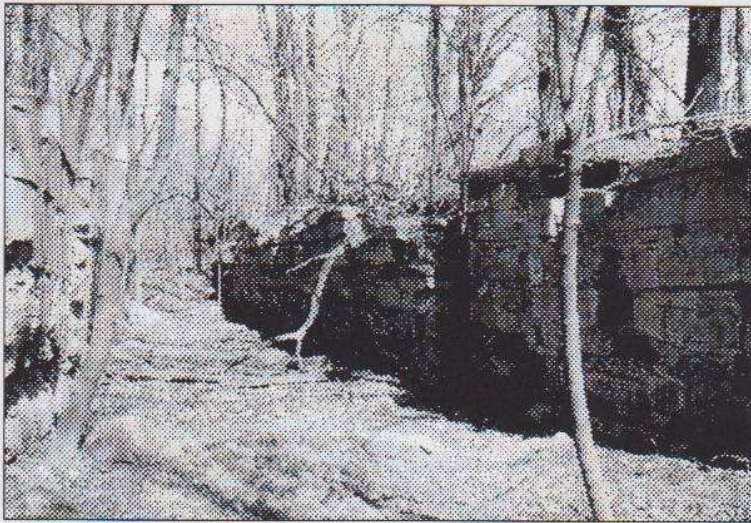
Fisher Lock No. 17 before it was buried. – Notebook III , p. 91
