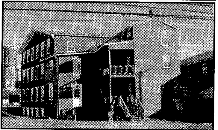
The Vinton House was built along the National Road. LG The Whitewater Canal basin was in the foreground. Products could be loaded/unloaded right into the Vinton House through the doors on the lower level. BS
