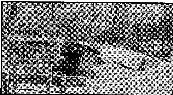
This 1873 Bowstring Arch bridge spans the restored Wabash & Erie Canal in north Delphi.
