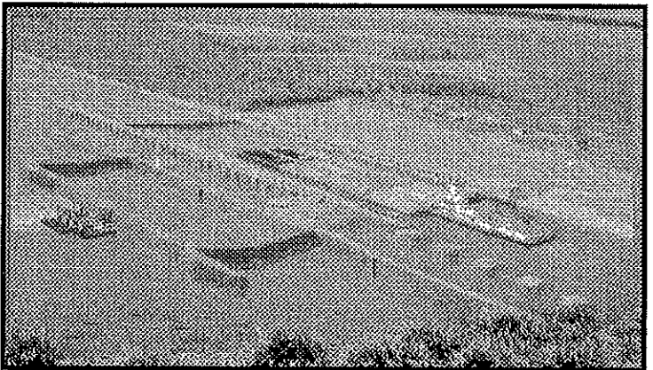
This mural depicts old Lock and Dam 52, which was a moveable wicket dam. In 1929 there were 51 similar structures on the Ohio River. It was 2,998 feet long, with upper pool of 302 ft. and lower pool of 290 feet. The lock was 110 feet by 1200 feet and the auxiliary lock was 110 feet by 600 feet. Photo -Bob Schmidt
