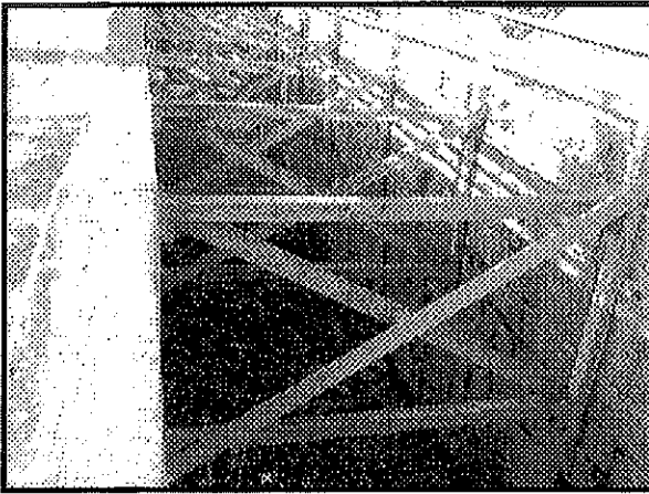
→ Lock #1 S has been braced for over 25 years. Plans are to repair it in the near future.
