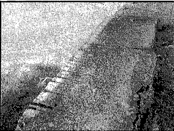
← Towropes have carved grooves into the stone on the lower end of the locks.
