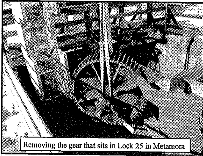
Broken gear shaft
