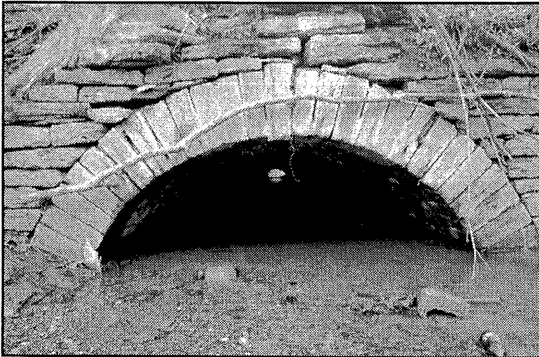
This Whitewater Canal stone arch culvert was recently located by Kim Ziegel, who is on the canal research committee for the Whitewater Canal and is from Covington, Kentucky. Photo - Kim Ziegel
