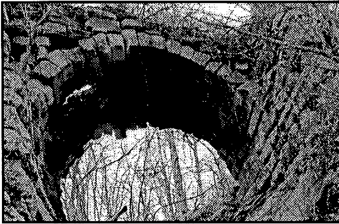
Olive Furnace arch had a gaping hole in it. LK
