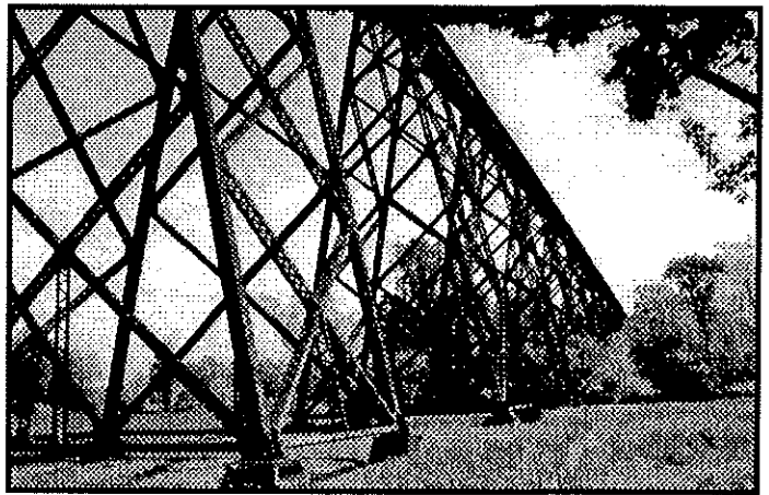
The Tulip Viaduct is one of the longest and highest trestles in the world. It is still in use. Photos by Bob Schmidt
