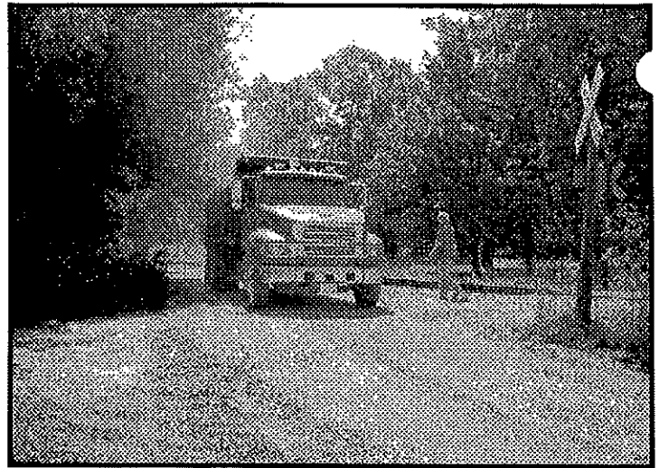
After trees and brush have been removed for the new trail, heavy equipment brings in and lays the gravel for the new trail. Note that the railroad tracks are atop the old towpath of the Whitewater Canal. Photos courtesy Mick Wilz
