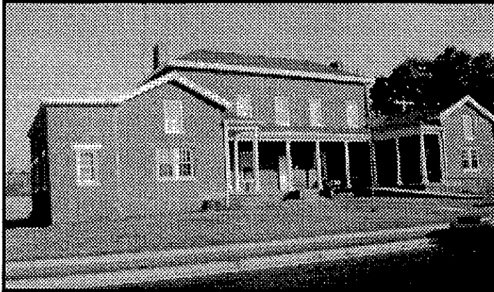
Front and rear views of the Vance-Tousey House in Lawrenceburg, Indiana, now on the National Register. Photos by Bob Schmidt
