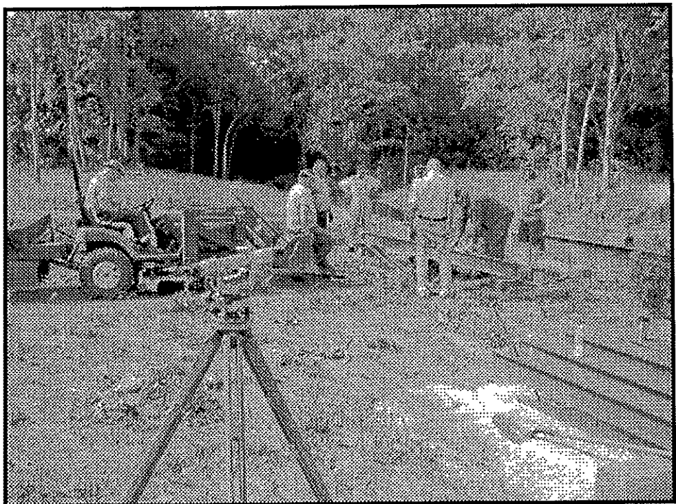
The 102-year-old 1905 Stearns Truss bridge from Medaryville has been restored and is being erected over the Wabash & Erie Canal at Delphi for use as a pedestrian trail bridge.
