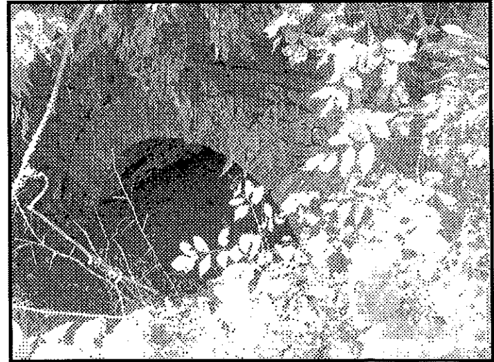
Possum Run Culvert has some stones missing on the side near the road and ugly stone covered with concrete has been placed between it and the concrete road culvert. Note that this face has had concrete added between the stones for stabilization. The culvert extends beneath the canal prism shown by the black line. The towpath is in the upper right hand corner of the picture with the bus. The opposite end of the culvert is in the lower right picture and has not had concrete added between the stones. Photos by Carl Bauer
