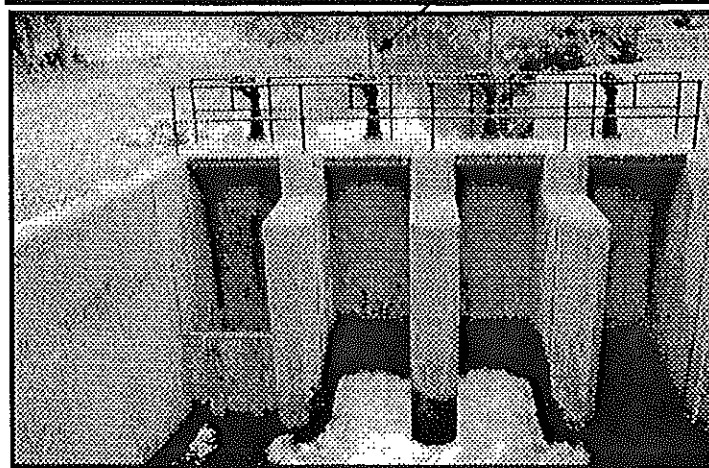
Just after the Delaware and Raritan Feeder Canal on the right releases excess water via a waste weir into the Delaware River on the left, sluice gates were built to protect the canal from flooding. Photos by Bob Schmidt
