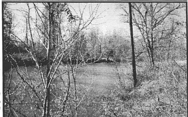
Below: The Wabash & Erie Canal at Francisco is a very good example of a watered canal prism. It is still about 40 feet wide, but probably is not four feet deep due to silt from nearby fields washing into it. A county road now runs along the towpath to the right of the picture. This section of canal would make an ideal place to canoe. Photo by Bob Schmidt
