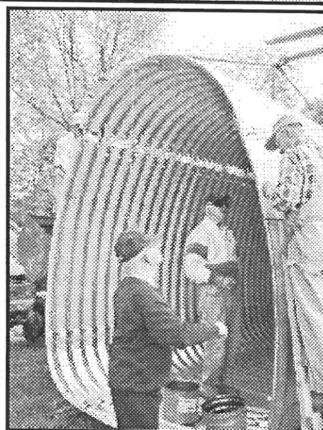
Carroll County Wabash & Erie Canal volunteers assemble a metal culvert for placement under an existing railroad track to connect two already completed sections of the Underhill Towpath Trail in Delphi, IN. Photos courtesy of Dan McCain
