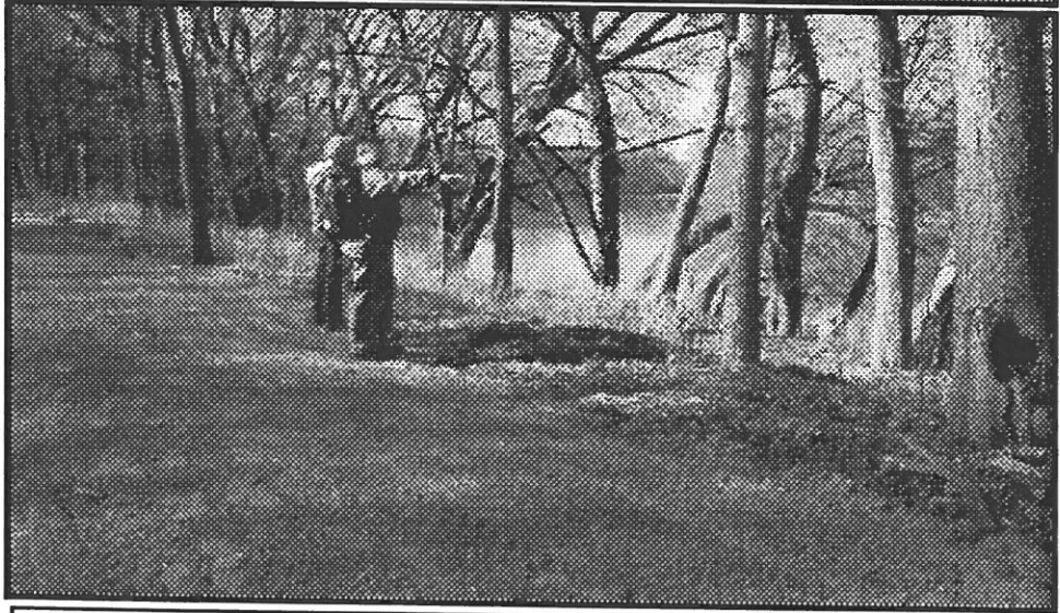
Top: The Interpretive Center's meeting room nears completion. Center: The drive to Campbell's ridge has material, which was once used to compact the Interpretive Center's foundation for several months, now placed upon it. Bottom: Boy Scouts look over the new trail they have built along the Wabash River. Photos courtesy Dan McCain
