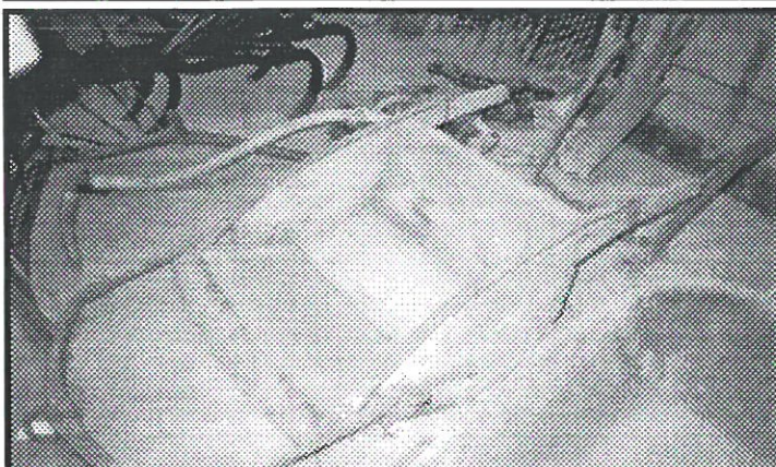
Slip scoop like those used to dig the canal
