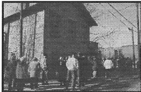
The Canal House built by John Brown in 1832 is used for Arts United offices today. Photo by Lynette Kross
