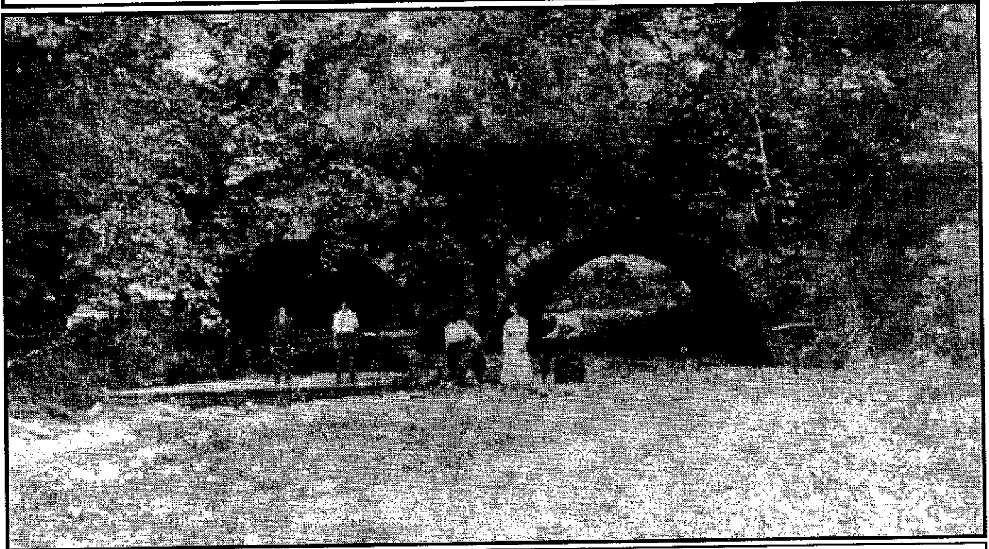
Above: This double arch stone culvert once carried canal boats on the Whitewater Canal across Yellow Bank Creek. Over the years this structure fell into disrepair and the state demolished it for safety reasons. They piled much of its rubble at the end of Yellow Bank Lock # 21. Historic Photo
