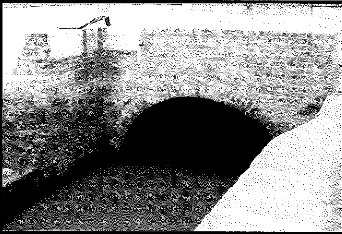
Top: Ft. Pulaski's Feeder Canal today with river in background. Bottom: The intake gate from the feeder canal into the fort's moat has a groove (not seen) where stop planks can be inserted to work on this structure.
