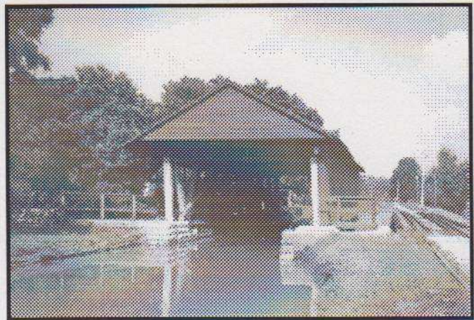
Duck Creek Aqueduct - Photo Bob Schmidt
