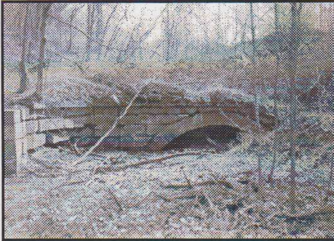
Cincinnati & Whitewater Canal Tunnel at Cleves, Ohio Photo - Bob Schmidt
