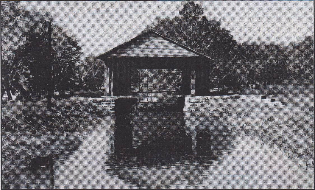
Looking through Duck Creek Aqueduct Photo by R. E. Stoops
