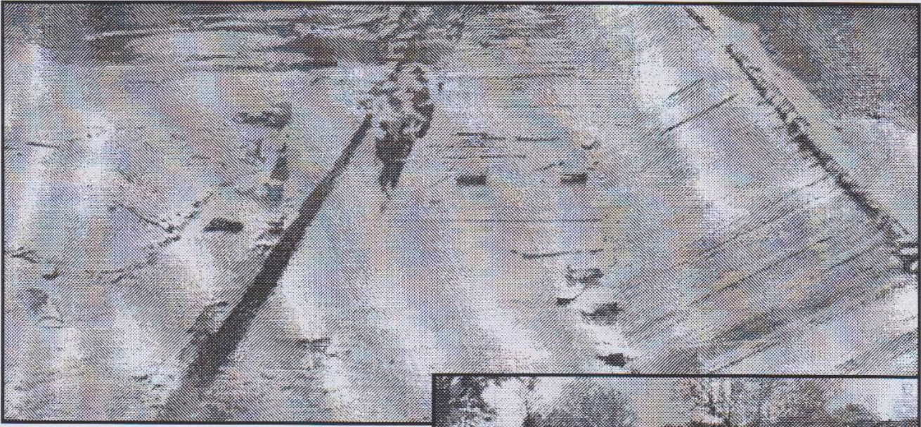
Above: The Laurel Feeder Dam is being repaired in the late 1800s after being breached as shown on the right. The dam is one of seven feeder dams along the original 76 miles of the Whitewater Canal. The wooden cribs were replaced by concrete, which later had to be replaced again. Below: The Laurel Feeder Dam pools water that is fed through this structure into the feeder canal and then to the Whitewater Canal. Fourteen miles of this early transportation system have been restored throughout the rolling hills of east central Indiana.
