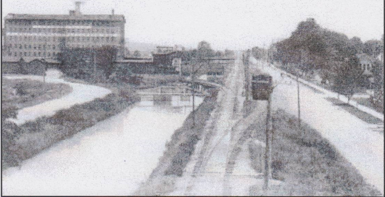
Looking north from 10th St. along Whitewater Canal at Connersville, Indiana E F Williams Photographer Connersville, Indiana
