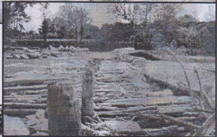
Above: The Laurel Feeder Dam is being repaired in the late 1800s after being breached as shown on the right. The dam is one of seven feeder dams along the original 76 miles of the Whitewater Canal. The wooden cribs were replaced by concrete, which later had to be replaced again. Below: The Laurel Feeder Dam pools water that is fed through this structure into the feeder canal and then to the Whitewater Canal. Fourteen miles of this early transportation system have been restored throughout the rolling hills of east central Indiana.
