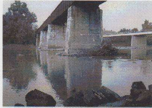
Railroad bridge across the East Fork of the White River looking to the north. The aqueduct that crossed here sat 42 feet above the water level and was 557 feet in length. The railroad piers sit where the aqueduct piers once stood. The Gil Hodges bridge is on the right on SR 57. Photo - R. Schmidt
