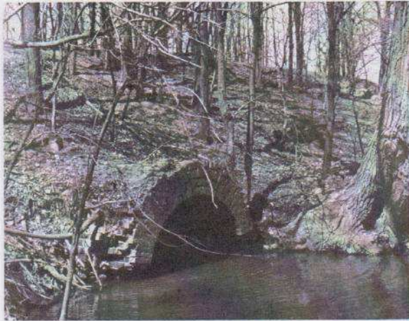
Simple brick culvert north of Lock 32 on T163.
