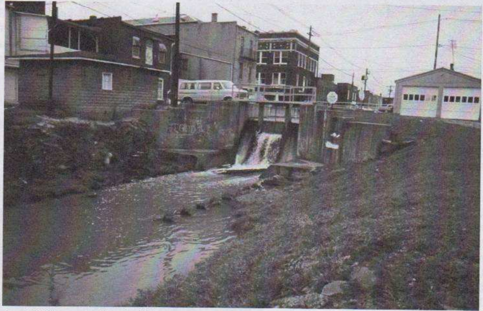
Lock 23N was replaced with a concrete dam and parts of the foundation timbers remain.
