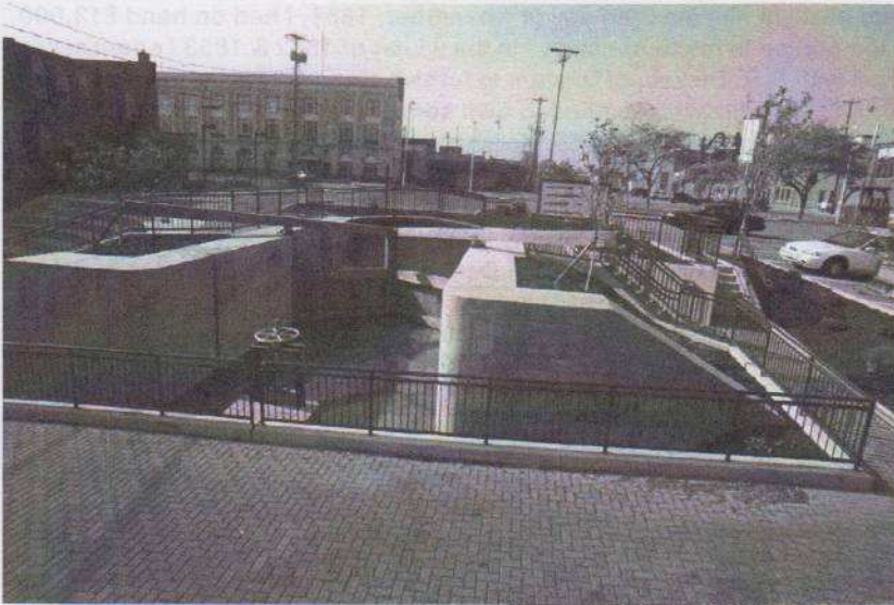
Lock 37 after renewal.
