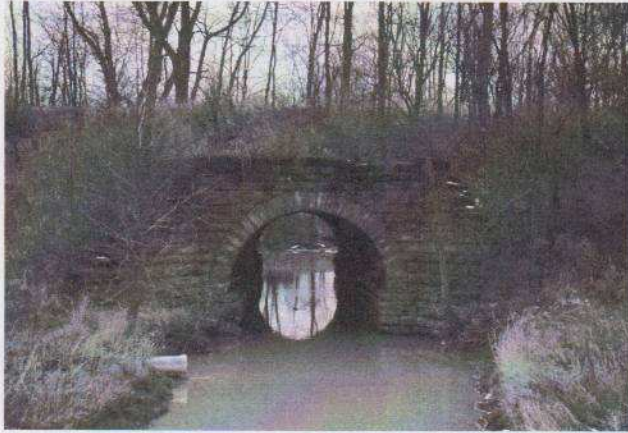
Flat Rock Creek Culvert, south of Junction on T163.
