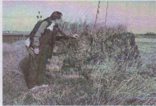
CSI President Bob Schmidt examines the remaining iron kiln from Paulding Furnace, on CR180, west of US127.
