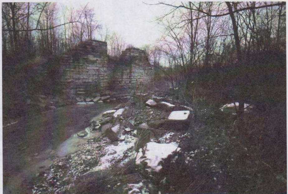
The Blue Creek Aqueduct was originally built without stone abutments and was 224 feet wide. It, and the Little Flat Rock Aqueduct, were rebuilt in 1859 with stone abutments. Today, only the north side remains. The south side was removed in the late 1950s.
