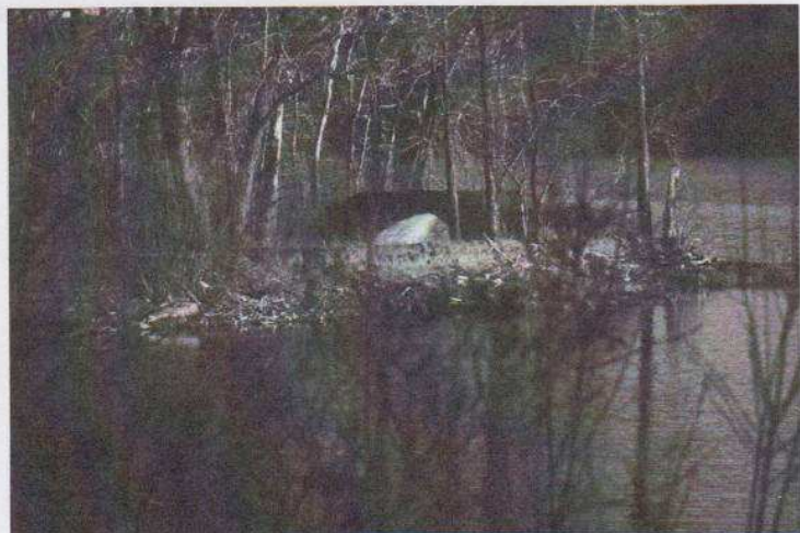
This small concrete bridge allowed mules to pass over a swale on the slackwater navigation, just west of Lock 40N where the boats entered the canal from the Maumee. A sign in the area says it was built in the 1930s by the CCC, but it clearly shows in the canal era plat maps.
