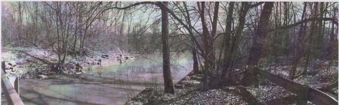
The Flat Rock Creek Aqueduct, which was removed by the CWA in 1934, was originally built without stone abutments and was 225 feet wide and built entirely of wood. It was rebuilt in 1859 with stone abutments and a 50 feet wooden flume.
