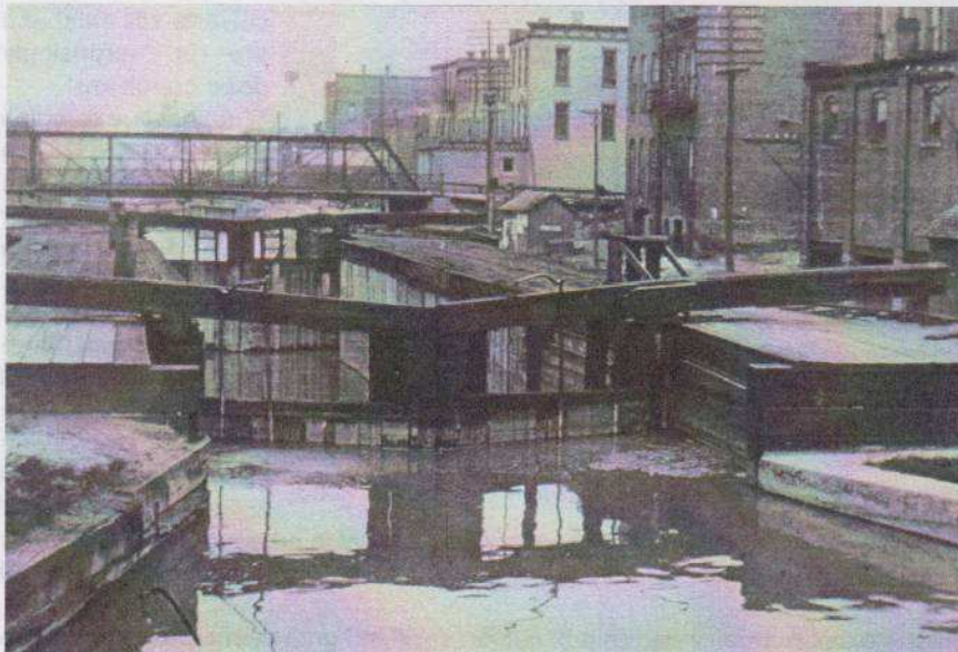
Typical wood lock (Lock 37Nin Defiance) lasted about 8 years.
