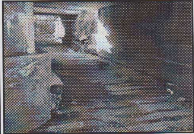
Culvert # 68 floor timbers at Daniel's Creek are seen in the top two photos taken looking south under Old US 24. The light shining down is between the road and the interurban bridge. The concrete and stone are parts of later structures. Photos by Kreig Adkins
