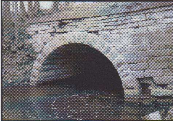
Stone arch culvert #73 at Prairie (LaFontaine's) Creek on Old Stone Rd. is seen looking north from the Wabash River on the right. On the left it is seen looking south. On this side the face stone, part of the stone culvert, the berm bank, and part of the bottom of the canal is gone. The foundation timbers are still in the creek bed. B. Schmidt
