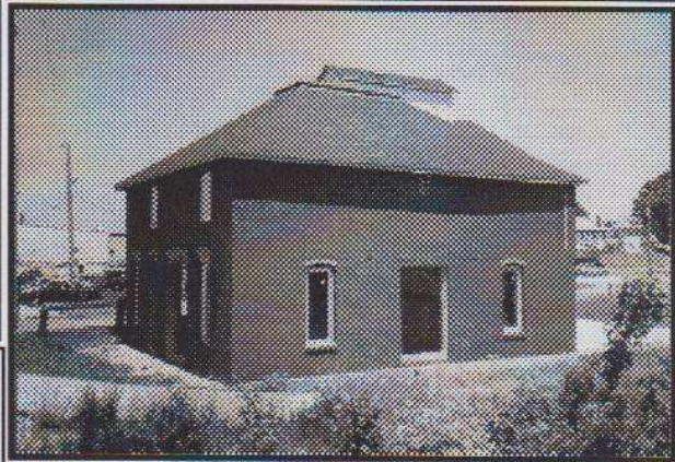
The Toll House, a square brick structure, was built in the late 1830s between the south side of the Wabash and Erie Canal and the Wabash River. It served as a toll house for the covered bridge that crossed the Wabash River. For many years George Dari operated a mercantile business here. Supplies and pioneers arrived by canal boat. It is the oldest historic structure in the town of Peru. Photo by Bob Schmidt
