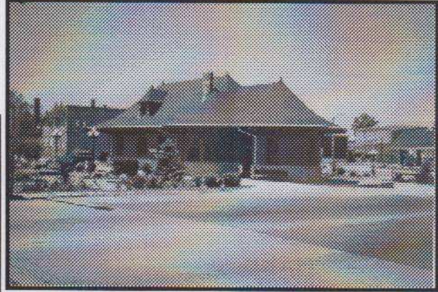
The C & O Depot was built in 1902 of limestone and brick and originally had a terra-cotta roof. Its cost of construction was $10,000. In 1991 the restoration of the depot with a garden addition was completed for $170,000. It is now rented for special events. Photo by Bob Schmidt
