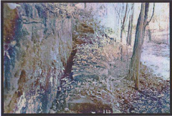
The cut away stone bluff has steps carved into it on the left, the canal prism has trees growing in it, and the Wabash River, which is located to the far right, is not seen. Photo by B. Migliore
