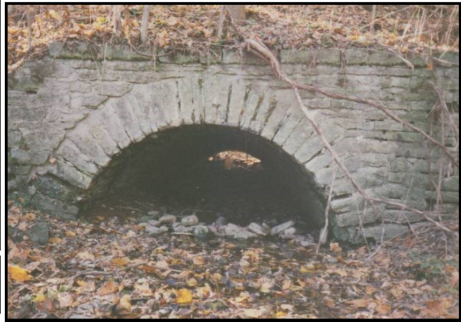
The Hagerstown Canal passed over this culvert and Nettle Creek passed through the arch. Photo by Bob Schmidt
