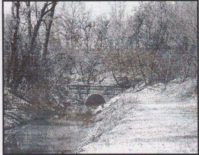
Delaware Creek Culvert
