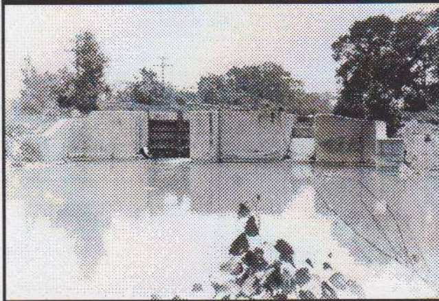
Concrete Lock 46 Toledo/Lucas County Public Library
