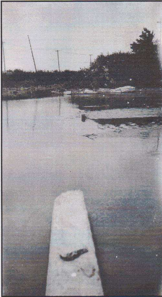
Maumee Power Company Intake With Weir At Entrance Canal flows north through upper end of picture Intake flows to right side of picture
