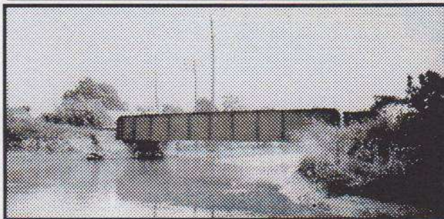
Nickel Plate Railroad Bridge Across Intake To Maumee Power Company
