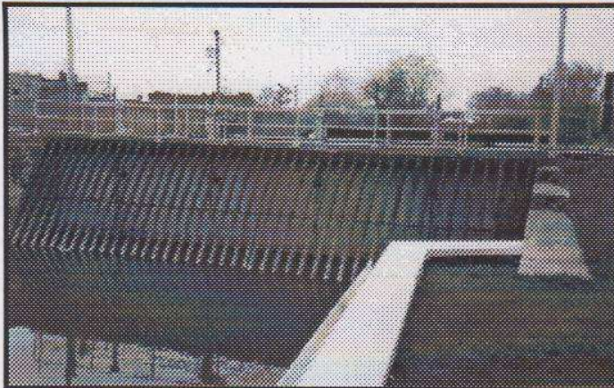
Water from the White River at Broad Ripple passes through this guard structure before entering the Central Canal and flowing toward the water treatment plant. Photo by Bob Schmidt
