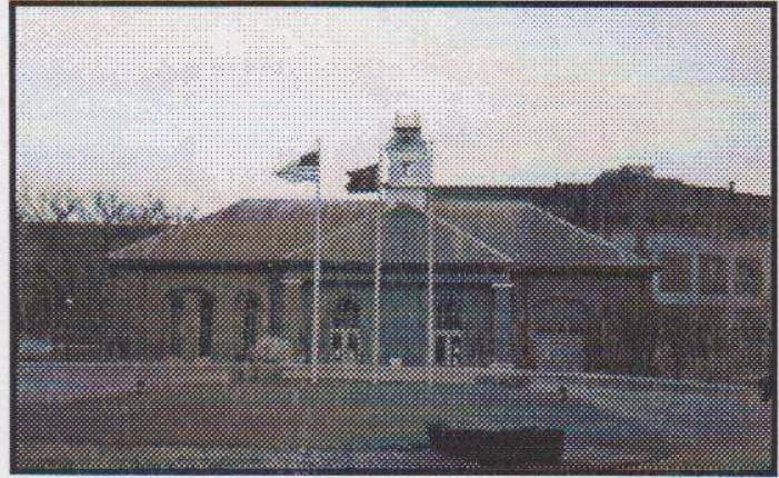
This pump house on West Washington Street was once operated using Central Canal water, which turned turbines to pump water from wells to Indianapolis water consumers. It is now used as a visitor center for White River State Park. Photo - Bob Schmidt
