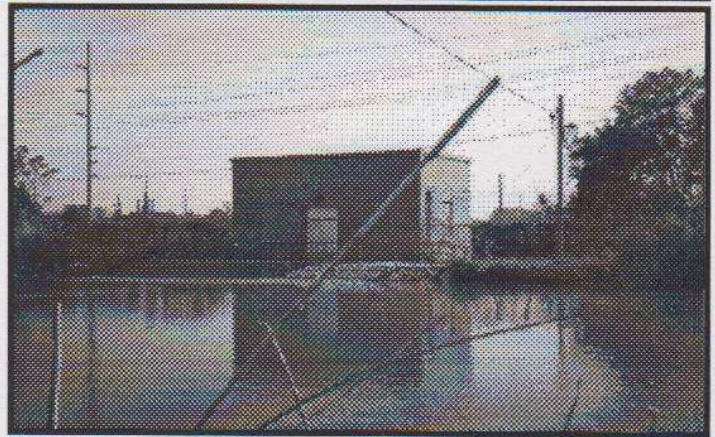
About 70% of Indianapolis' water supply is taken from the Central Canal at this intake site and treated in the purification plant in the background. Photo by Bob Schmidt
