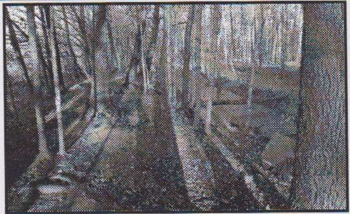
The Central Canal towpath and prism north of Indianapolis, Indiana, is overgrown by trees today. Photo by Chuck Huppert
