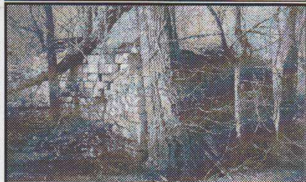
Below: A closer view of the above abutment. Note how time, ice, and roots are pulling the stones apart.
