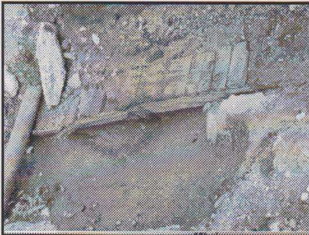
Above: Some of the timbers that were used in building the cribs still had bark intact on them. Below: The top of the cribs were covered with planking.
