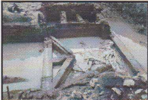
MITRE SILL AS FOUND IN THE GRONAUER LOCK IN NEW HAVEN INDIANA
