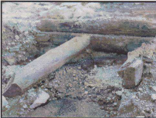
Above: Some of the timbers that were used in building the cribs still had bark intact on them. Below: The top of the cribs were covered with planking.
