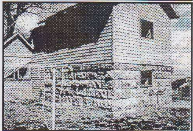
Below: The "Warm House" of Dr. James M. Boyd of Annapolis, IN. The stone walls were formerly a part of the Rockport Mill race. Photos by Charles Davis 2000
