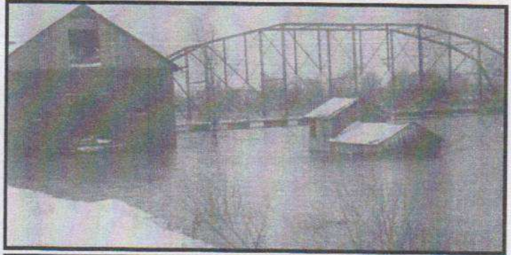
This 1913 photo shows the Wabash River at flood stage at Montezuma. The large building at the left was a warehouse and sat astride the Wabash & Erie Canal so that boats could enter and be loaded and unloaded inside. Here the canal prism is under the flood waters.
